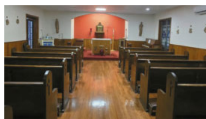
Renovation of the Convent Chapel
